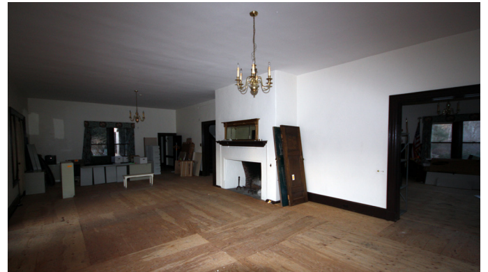
While much of the interior finishes are in fair condition, selective restoration to the floors and fireplaces would be recommended at the main house.
