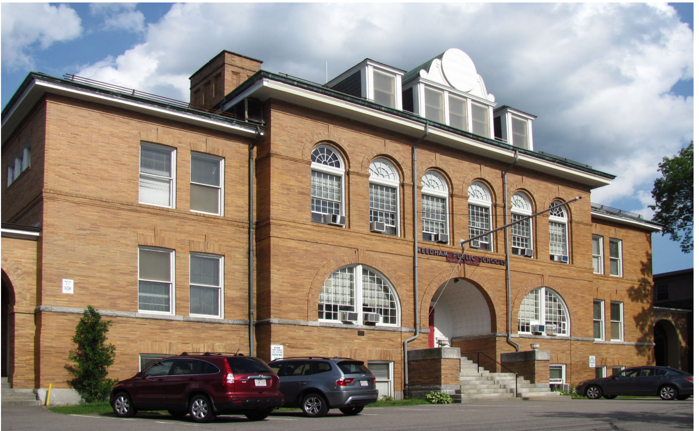
EXISTING EXTERIOR CONDITION
